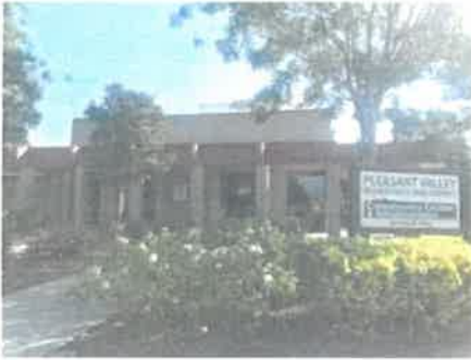
Photograph 1. View of the Administration building located on the subject property, facing northwest.
