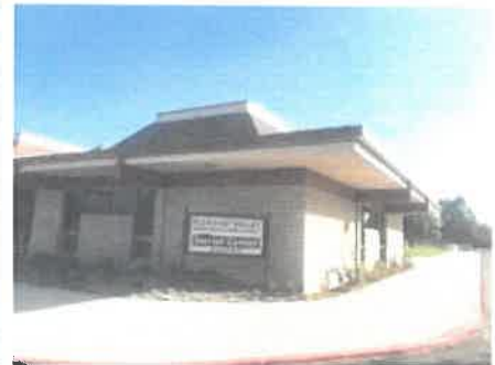
Photograph 3. View of the Senior Center Building, facing north.
